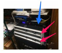
In the liquor storage room, turn on the amplifiers (red arrows on left photo) and verify that the speakers are not muted (unit above amplifier shown by blue arrow - has 6 small buttons on lower right - they turn red when muted - we do NOT want red lights!!)
